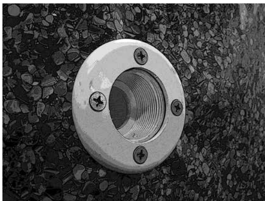
Return faceplate installed.
