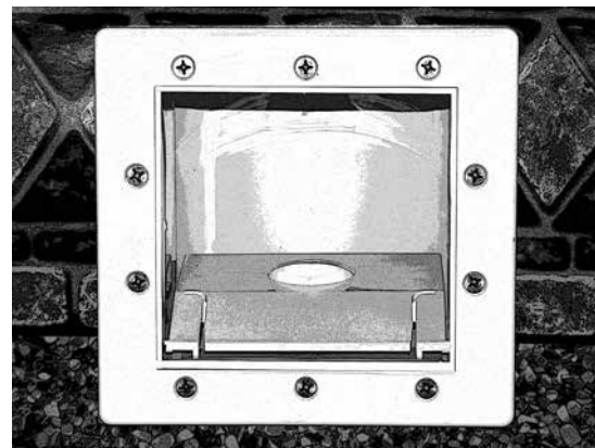
Skimmer faceplate installed.
