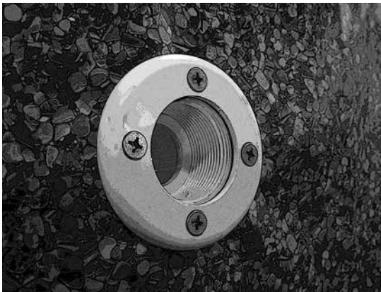
Return faceplate installed.
