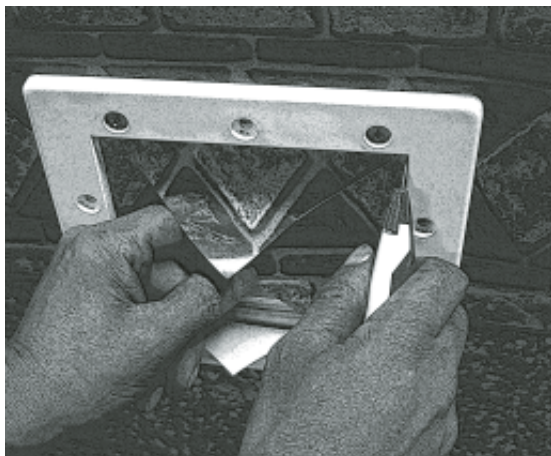
Trim liner from skimmer opening.
