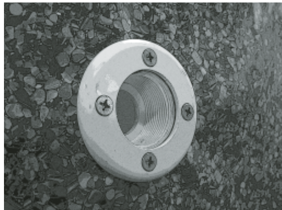
Return faceplate installed.
